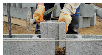
Chantier Vertical Bloc® © Guy Yoyotte
